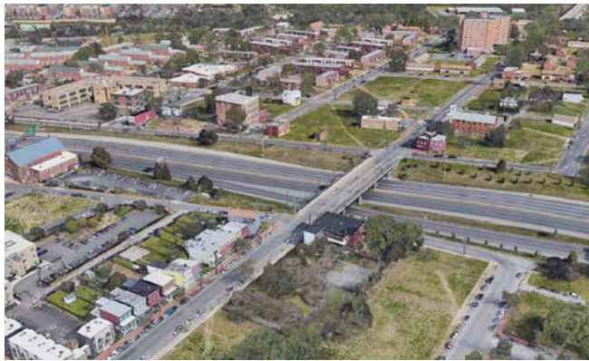
EXISTING GILPIN COURT PUBLIC HOUSING Richmond, VA
